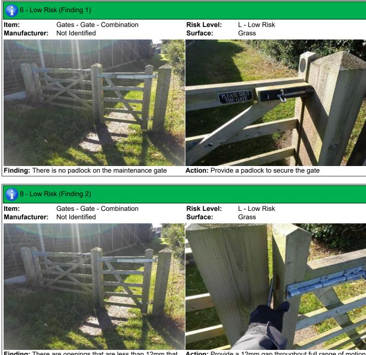
**Finding:** There are openings that are less than 12mm that could trap or crush fingers
