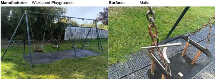
Finding: The chain openings are in excess of the 8.6mm as Action: Monitor - No remedial work recommended recommended by BS EN 1176
