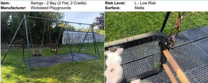
Finding: There are caps missing from the underside of the Action: Replace missing caps under the seats seats
