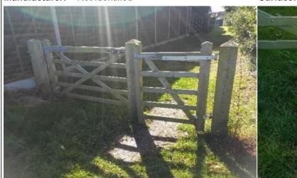
**Finding:** The area under the gate has eroded leaving uneven areas, or the concrete foundations exposed, resulting in trip hazards at the entrance/exit to the playground
